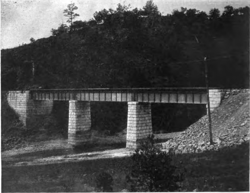
Bridge across the Pichachic Arroyo.
